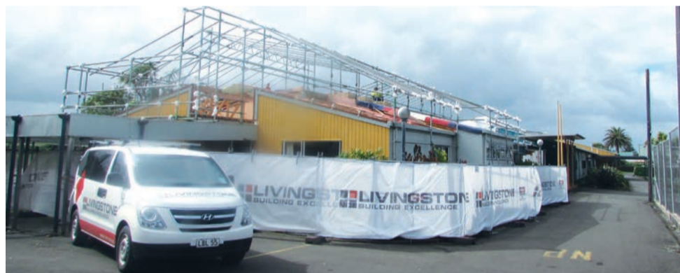
Reroofing work at Opunake High School was laid bare after strong winds last week.
